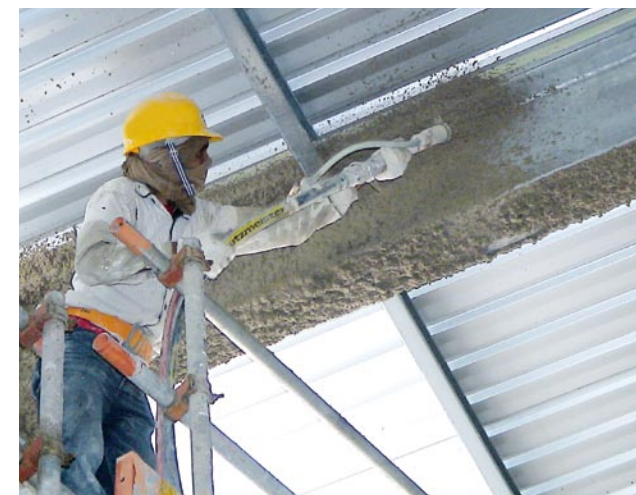
...or for special applications, seen here being processed as fire-proofing mortar.
