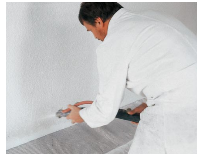
Worm pumps type S 5 and SP 5 can be used for all pumpable mortars up to an aggregate grading of 6 mm, whether as normal base coat plaster (large picture), as a decorative texturing plaster...
