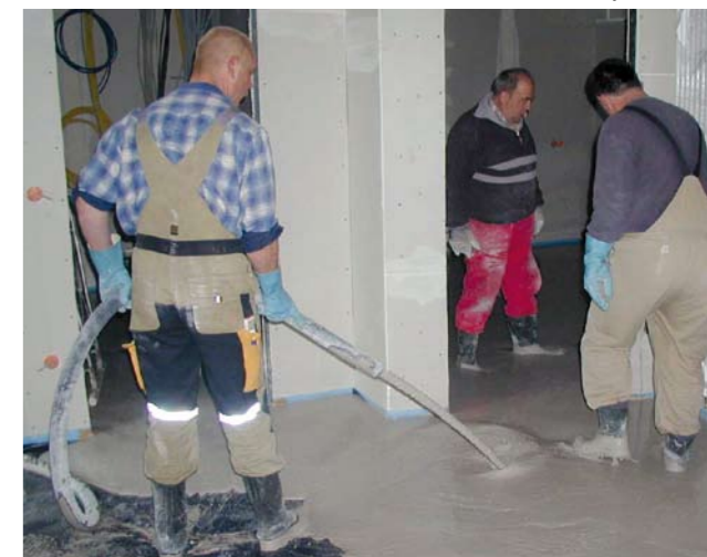
Also self-levelling screed can be placed from a long distance.
