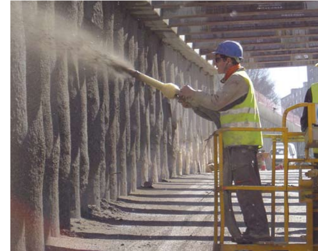
Concrete pumps, like this P 715, are a part of the wide range of systems. They can be used for placing shotcrete, ...
